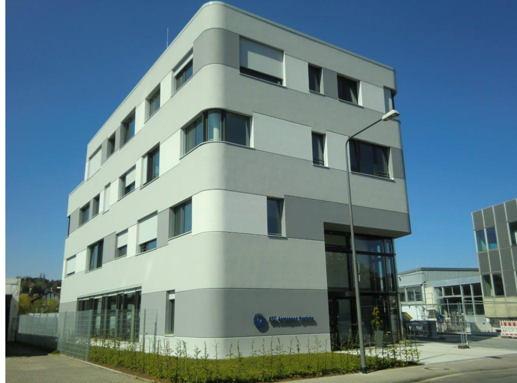
Nord-Micro Datacenter local side Germany/Frankfurt
