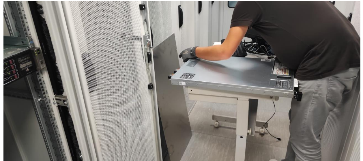
Preparation of Datacenter Components
