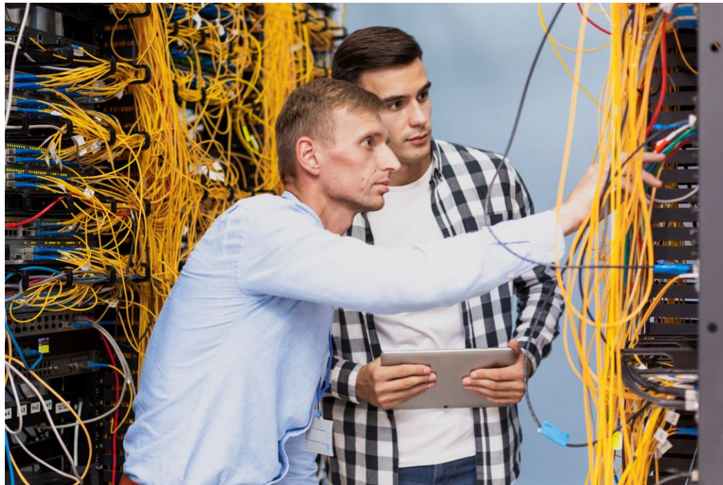
Datcenter local side UBS Bank in Germany/Frankfurt
