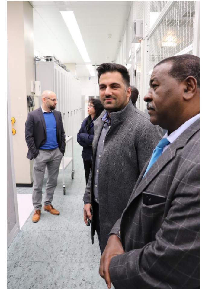
GGSC Partner Diamond in UZH Datacenter
