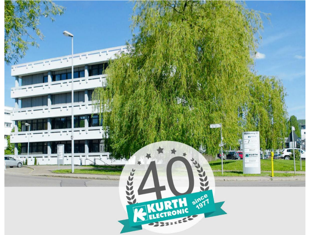
Kurth Electronic Headquarter Nürnberg/Germany
