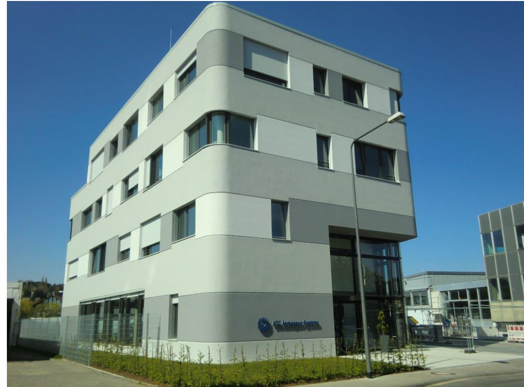
Nord-Micro Datacenter local side Germany/Frankfurt
