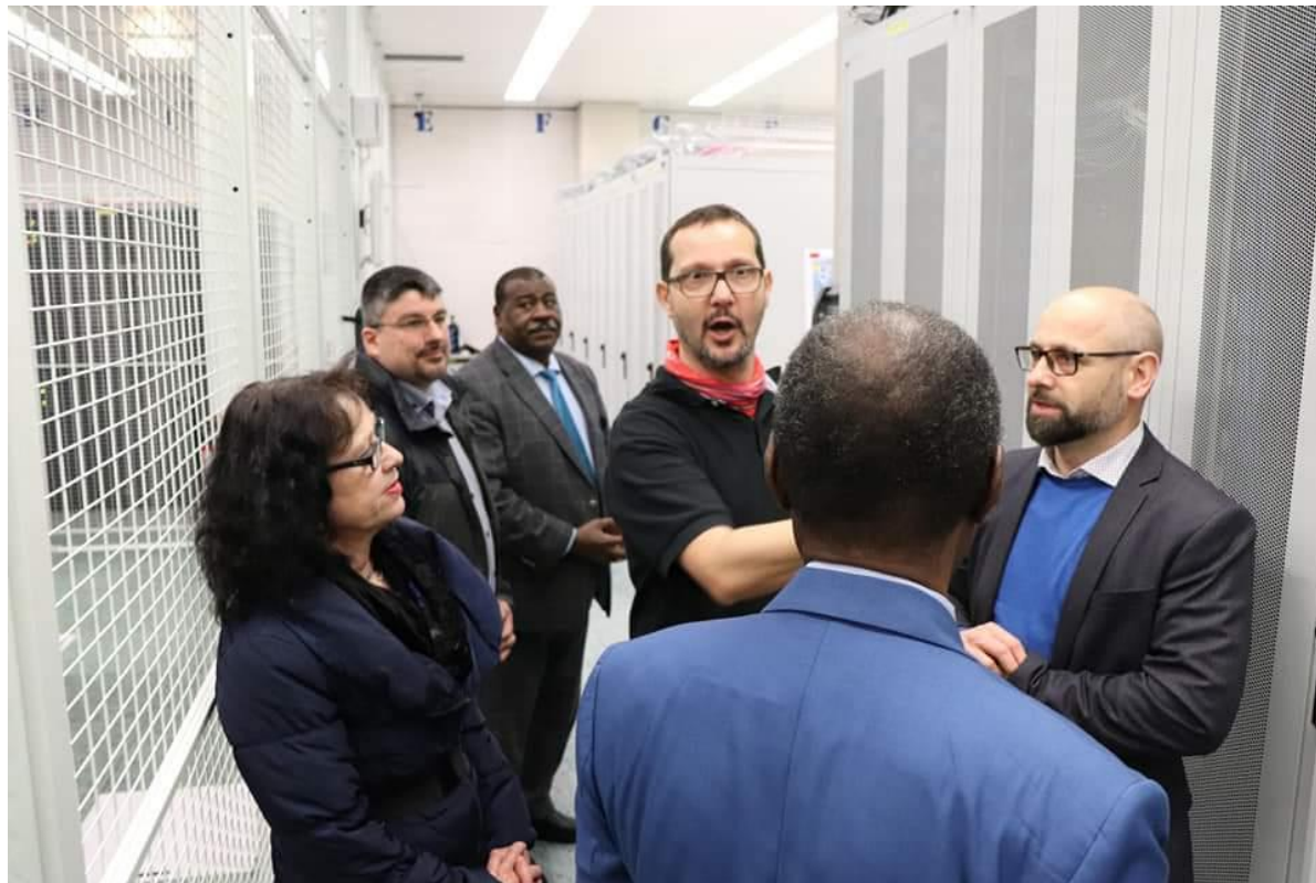
GGSC Partner Diamond in UZH Datacenter
