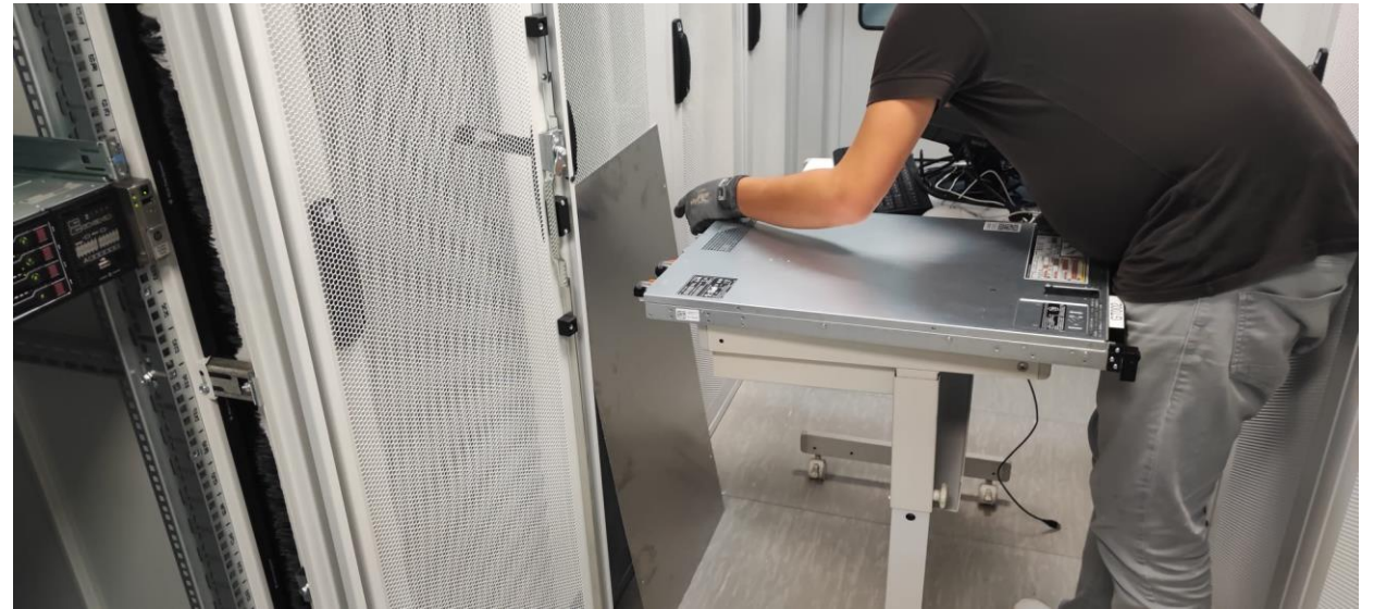
Preparation of Datacenter Components
