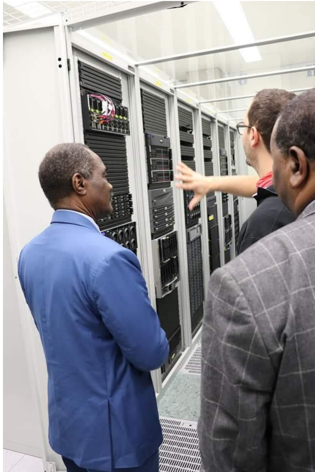
GGSC Partner Diamond in UZH Datacenter
