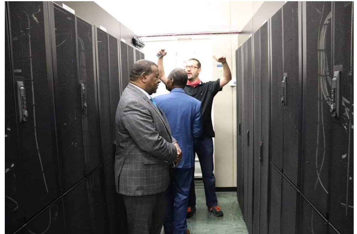
GGSC Partner Diamond in UZH Datacenter
