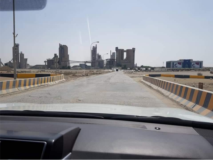
Gulf Cement Factory Construction Site in Doha
