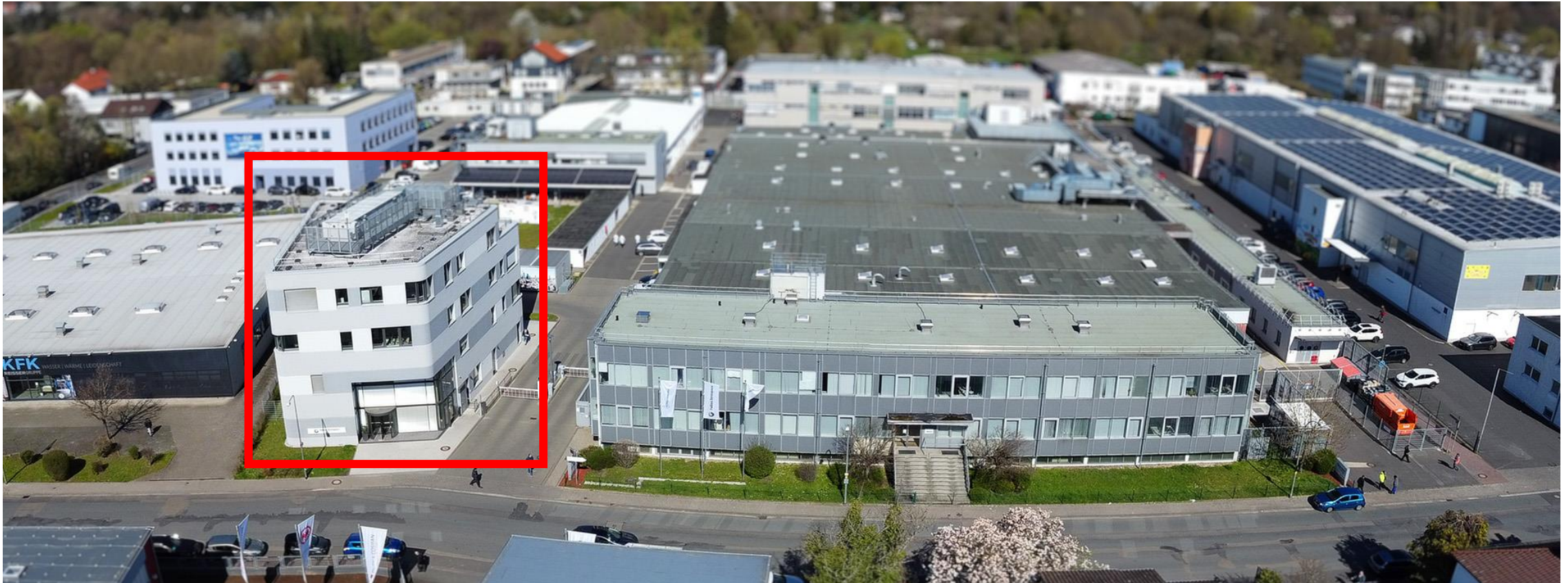
Nord-Micro Datacenter local side Germany/Frankfurt
